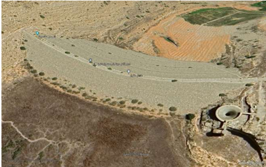
Figure 1: shows Bou Mansour Dam prior to its collapse
