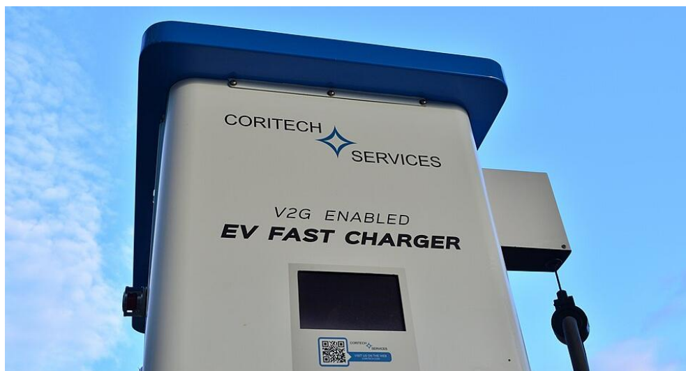
Figure 3 A vehicle-to-grid (V2G) capable fast charging station. Such bidirectional chargers allow EVs to both draw power from and supply power to the grid. (Source: Wikimedia Commons, CC0)
